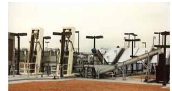
Left: Two new Inkos bar screens discharge screenings into a triple-inlet, Inkos shaftless screw conveyor. Located in a Seismic Zone 4, this project also includes a Inkos shaftless screenings washing press. The press, located at a lower level, receives screenings from the conveyor by means of a flexible connecting chute. There is a centrally located inlet on the screenings conveyor that provides for a future Inkos model SRP bar screen.
