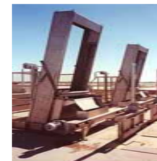
Left: Two new Inkos bar screens discharge screenings into a triple-inlet, Inkos shaftless screw conveyor. Located in a Seismic Zone 4, this project also includes a Inkos shaftless screenings washing press. The press, located at a lower level, receives screenings from the conveyor by means of a flexible connecting chute. There is a centrally located inlet on the screenings conveyor that provides for a future Inkos model SRP bar screen.
